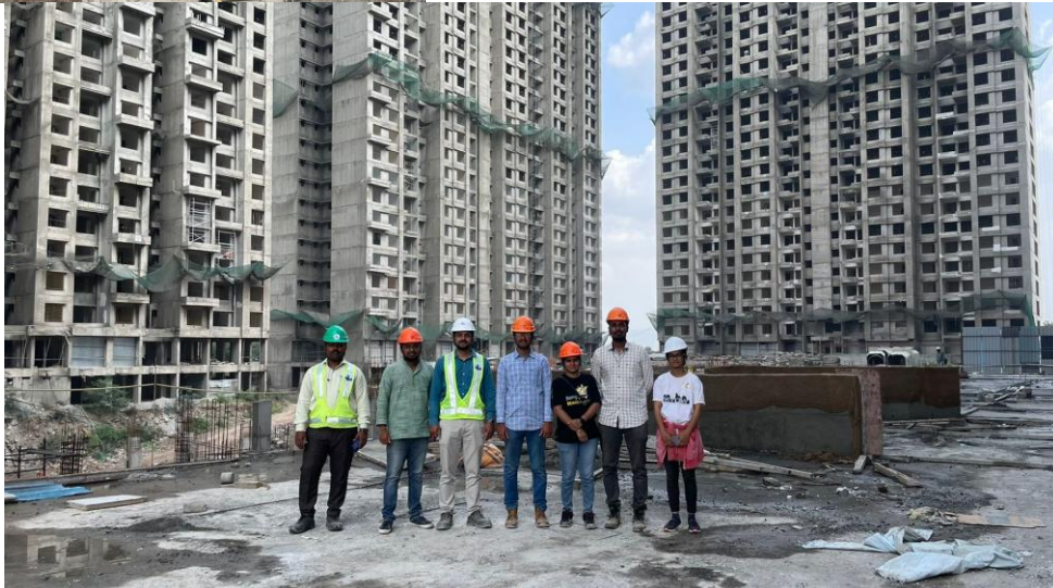
M.Arch Students engaged in on-site learning and assisting the project team at the VTP Euphoria Project Site
